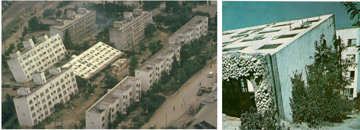
Fig. 1.5 Building tilt and settlement due to liquefaction during 1964 Niigata Earthquake ( click for earthquake )
