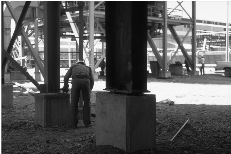
Figure 2.31 Earthquake-induced foundation settlement (Michoacán Guerrero earthquake, 1985).
