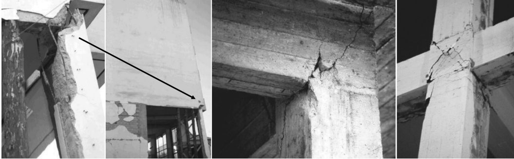
Figure 2.21 Shear failure of beam–column joints.
