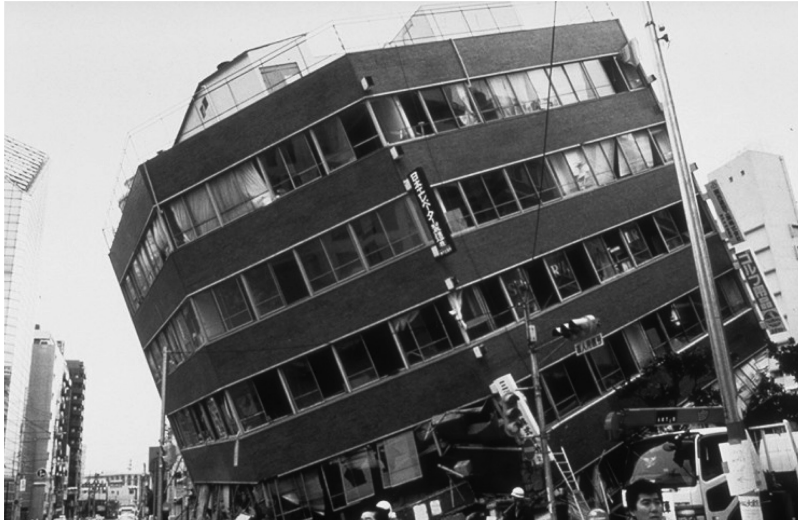
Figure 2.28 Bearing capacity failure due to liquefaction (Hyogo-ken Nambu earthquake, 1995).
