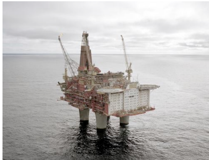
Figure 2.12 Concrete Gravity Statfjord B platform [H. Tonneson and F.H. Sandberg, 1983. Statfjord B Platform].
