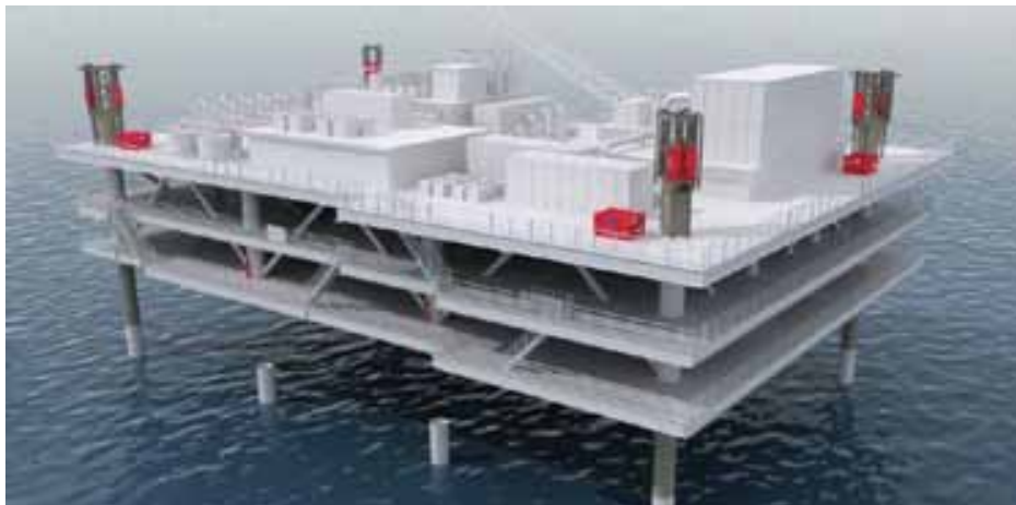
(iii) Details of modular assembly in the top deck and two cellar decks of the steel jacket structure. (Technical brochure, Offshore, ALE. www.ALE-HEAVYLIFT.COM ,)
